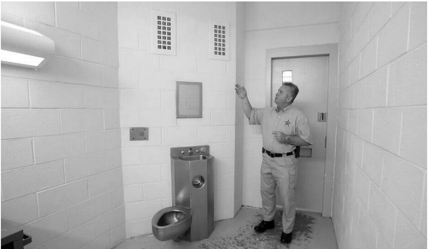
Durham County Sheriff Mike Andrews discusses the old grates in jail cells which are being replaced with new “suicide proof” vent grates in a wing of the Durham County Detention Center Monday, June 6, 2016. A section of the jail is being renovated to accommodate mentally ill prisoners. Chuck Liddy cliddy@newsobserver.com
